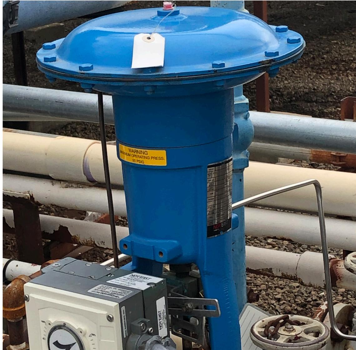
**NEW CONTROL VALVES:** The new valves are “Control Valves” which are integrated into the controlled automation system. This new automation makes the terminal safer and more efficient.
